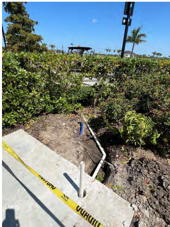
Pipe stubbed out for water fountain.
