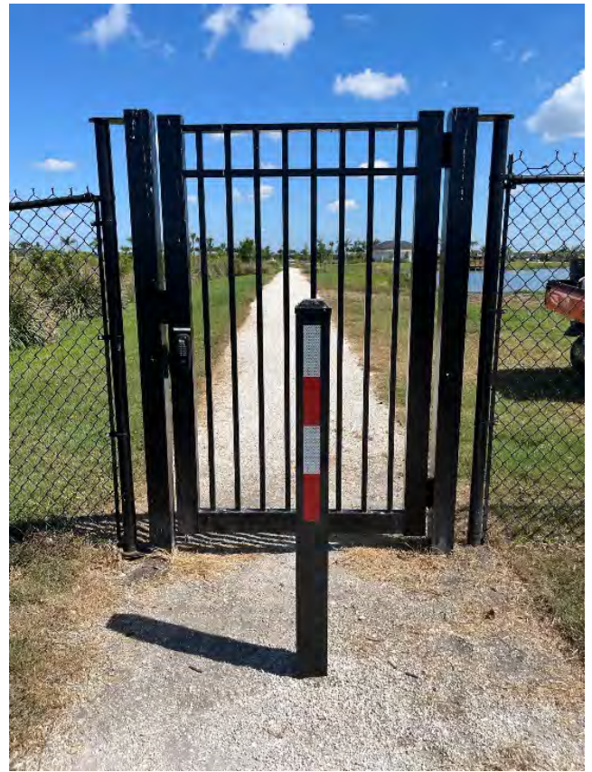
New barrier placed along path.
