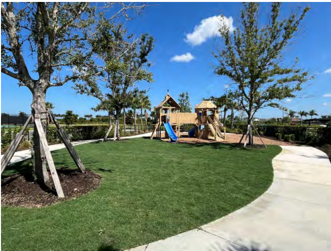
Turf installed on playground.
